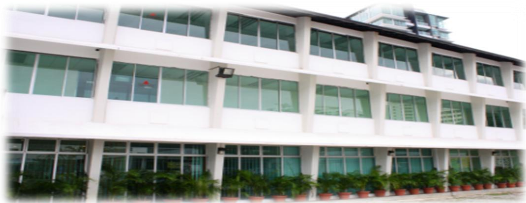
Block D, ICRI Campus Exterior – Ground Level
